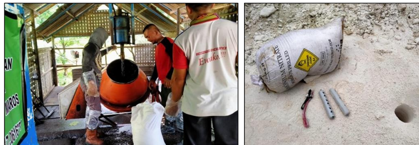
Figure 3. Mixing of the explosives used
