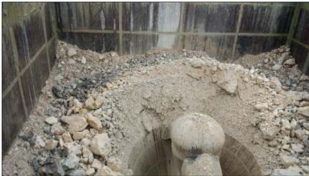
Figure 8. Rock Fractionation in the Hopper Crusher
